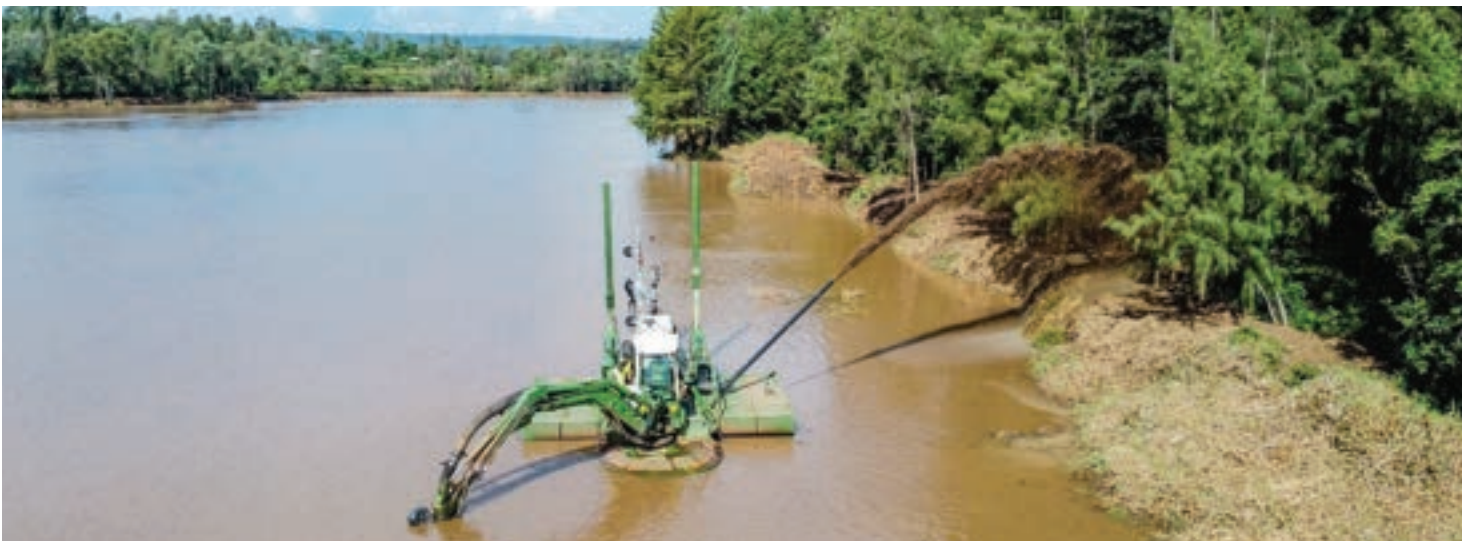
Desilting using the suction pump
